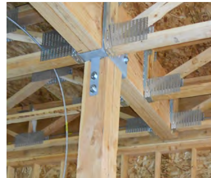
Figure 34: Beam-Column Connection
