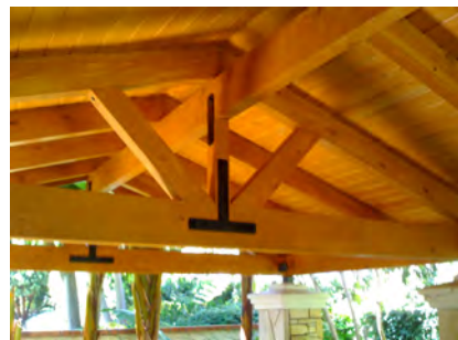
Figure 11: Type IV Construction
