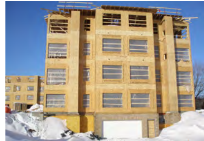
Figure 10: Type V Construction
