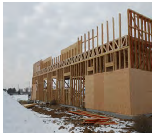
Figure 38: Wall Bracing
